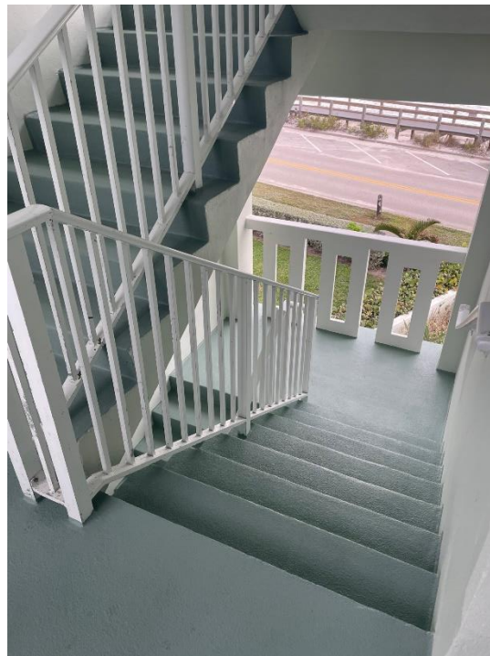
Pic 6 – East stairwell
