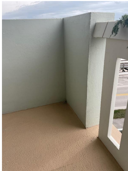
Pic 8 – Typical limited access balcony guardrails
