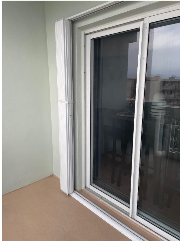
Pic 9 – Typical limited access balcony sliding glass doors w/ shutters
