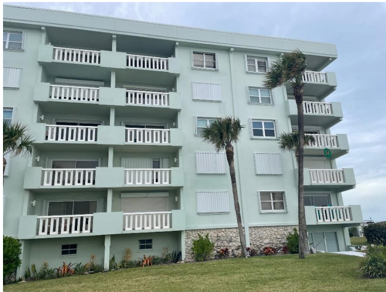
Pic 10 – Limited access balconies at the south elevation
