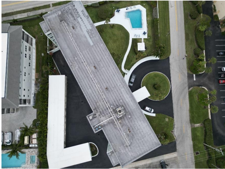
Figure 1 – Aerial view of structure
